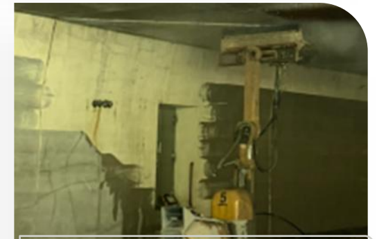
Concrete removal robot
